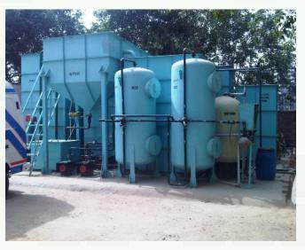
MBBR - (Moving Bed Biofilm Reactor): This process is based on the aerobic biofilm principle and utilizes the advantages of activated sludge and other biofilm systems without being restrained by their disadvantages. The basis of the process is the biofilm carrier elements that are made from polyethylene which provide a large protected surface area for the biofilm and optimal conditions for the bacteria culture to grow and thrive.
